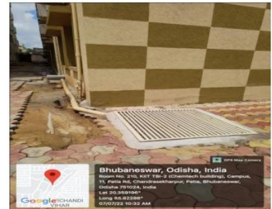
Rainwater Recharge Pit
