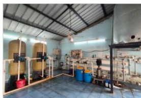
Central R.O. Based Water Treatment Plants
