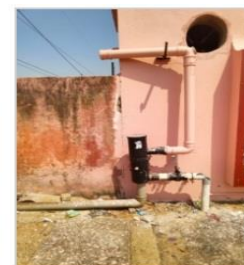
Rainwater Harvesting Equipment (Location – 3)
