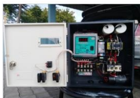
Automatic Water-Level Controller For Over Head Tanks
