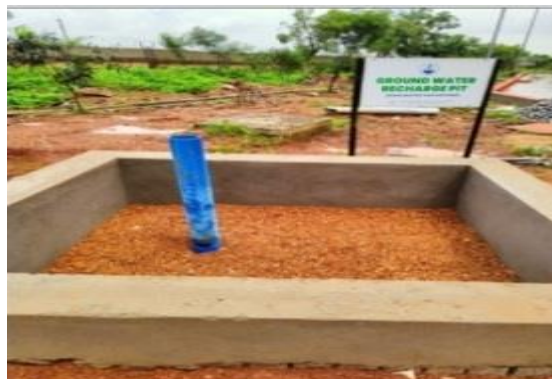
Ground Water Recharge Pit – 2
