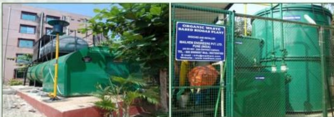
Figure 10. Organic waste based Bio-gas generation plants placed at the campus.
