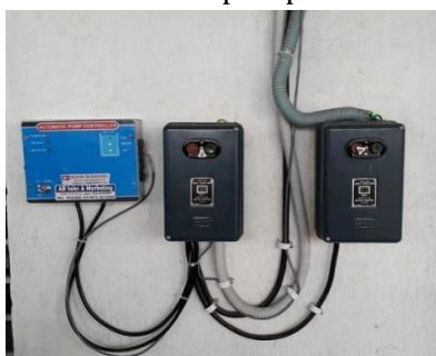
Automatic Water Controller with Pump Starter
