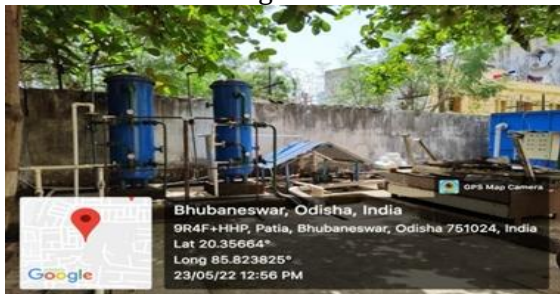
STP at Campus 18 (Capacity – 90 KLD)
