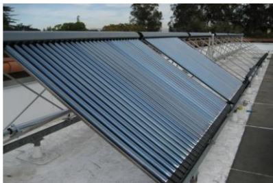
Solar Water Heating System
