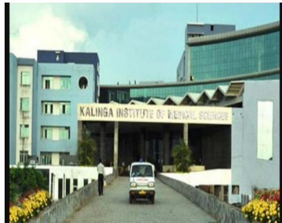
Fig. 3.1: KIMS Hospital, Bhubaneswar
