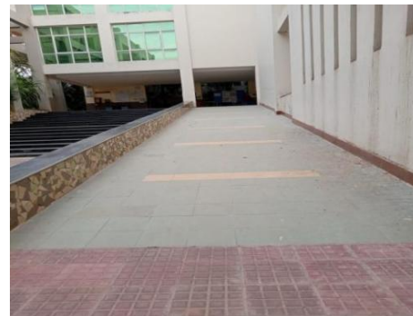
Fig. 7: Ramp for wheelchair users
