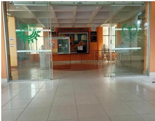
Fig. 5: Automatic Sliding Doors
