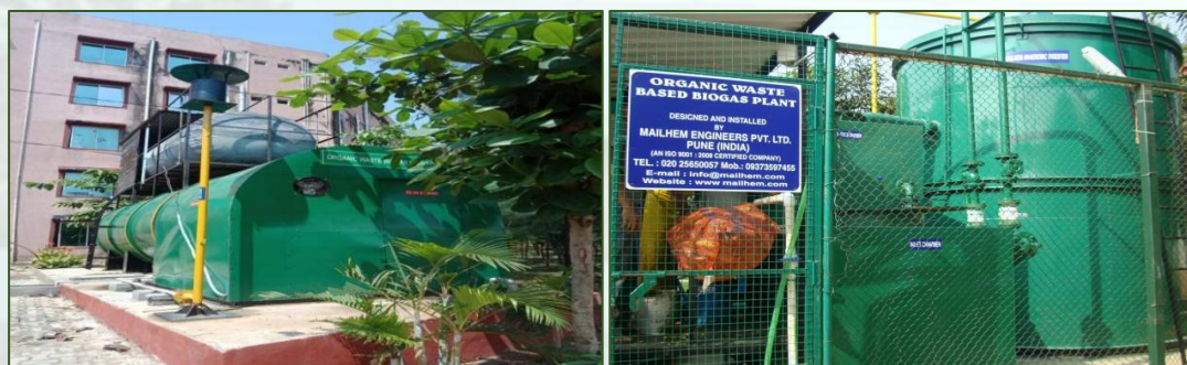
Figure 10. Organic waste based Bio-gas generation plants placed at the campus.
