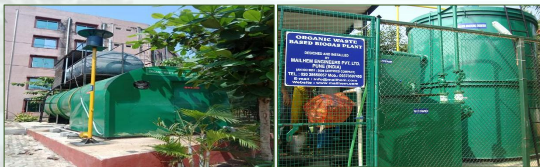
Figure 10. Organic waste based Bio-gas generation plants placed at the campus.
